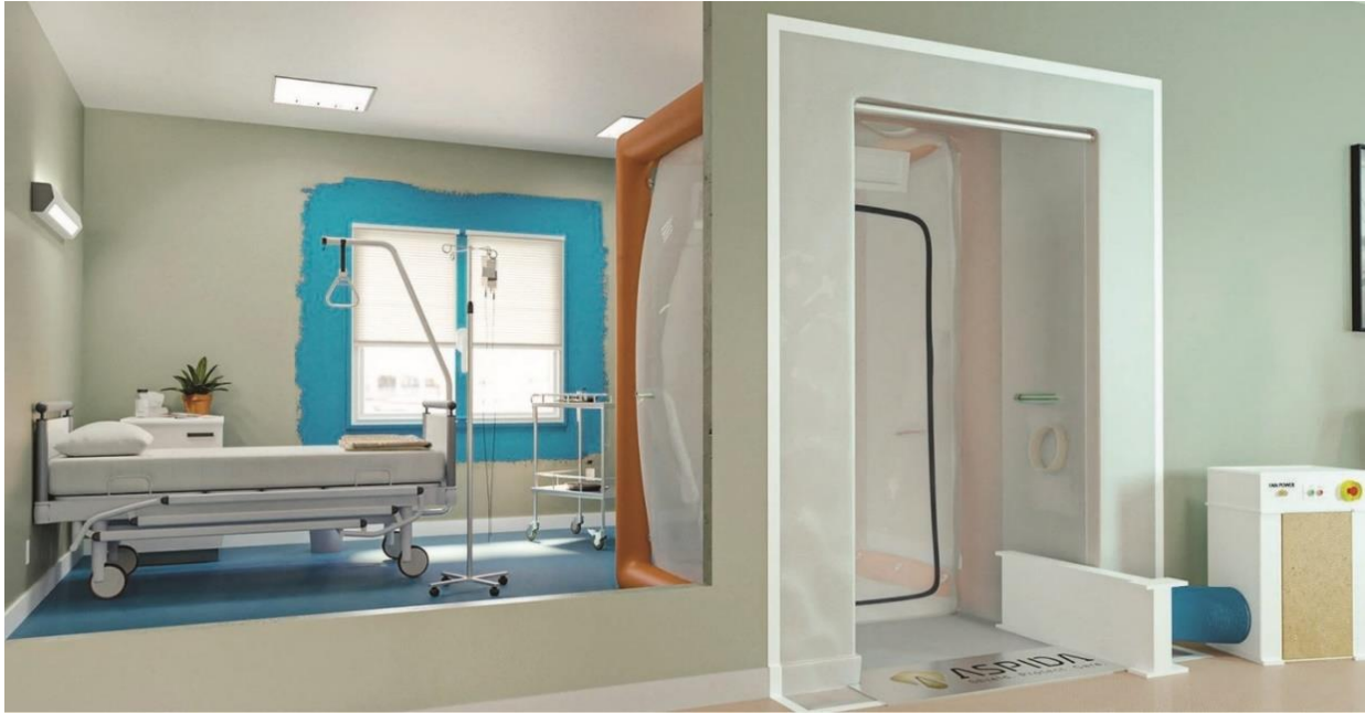
Fig. 4 Remodeling existing rooms into contagion isolation rooms
